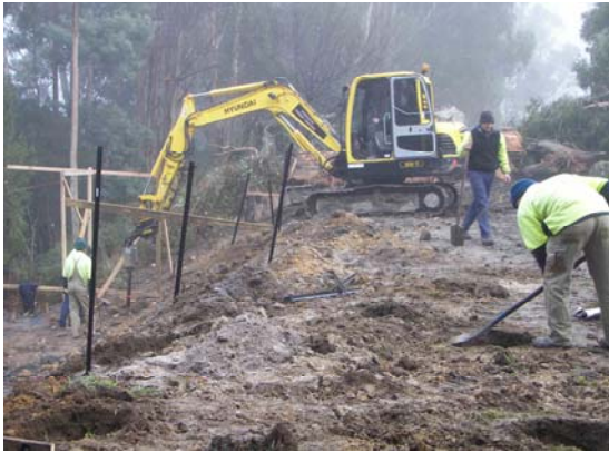
Work began recently on construction of the Upper Huon Community Centre
