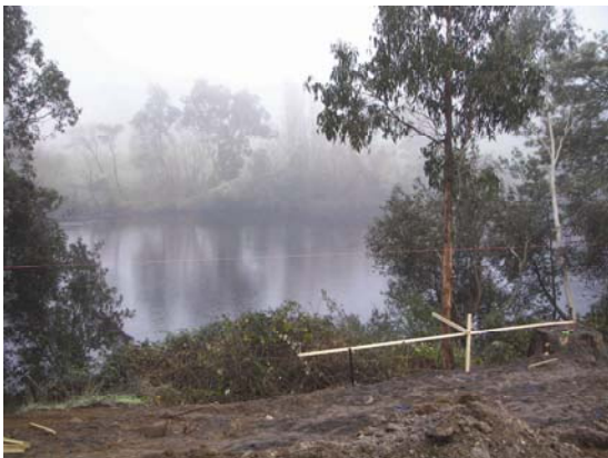
The new Upper Huon Community Centre will offer uninterrupted views of the Huon River from the centre's open air deck
